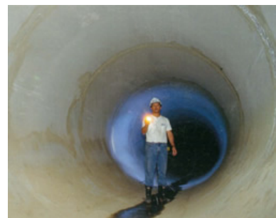
Inspection of completed Cast-In-Place Concrete Pipe.
