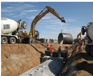
120" Cast in Place.
