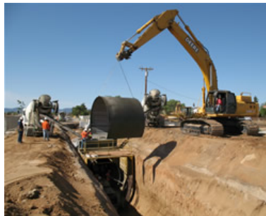
Cast in Place.
