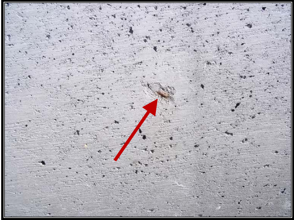
Figure 4-9. Exposed Cage Spacer – Acceptable
