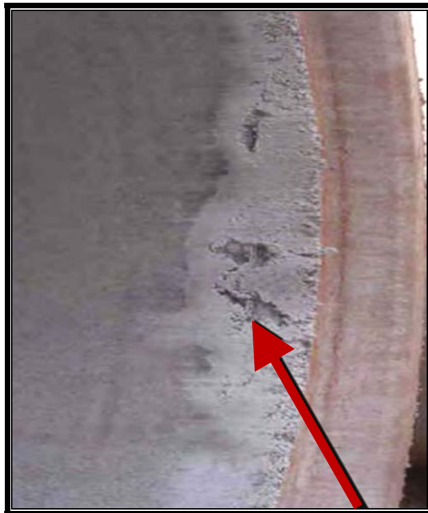
Figure 3-3. Honeycombing – Repairable
