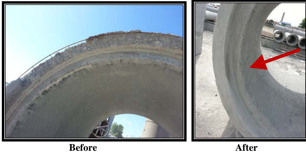
Figure 2-10. Plant Bell Repair - Acceptable
