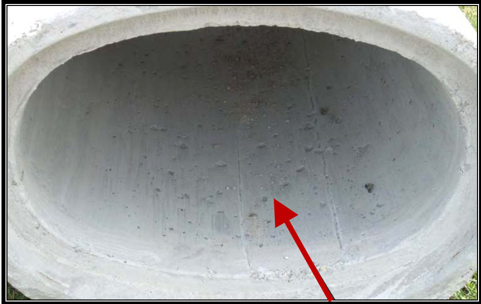
Figure 3-4. Bug Holes and Shallow Pitting – Acceptable
