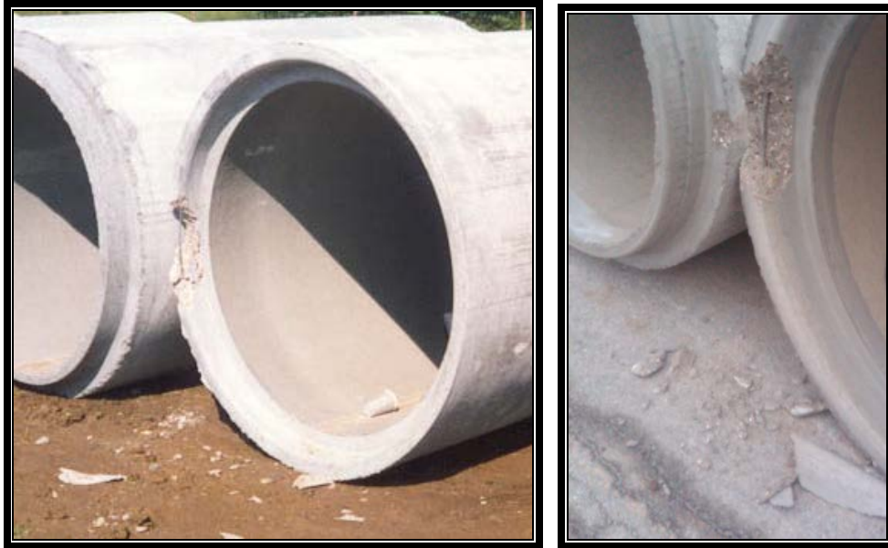
Figure 2-8. Shipping and Handling Damage – Repairable
