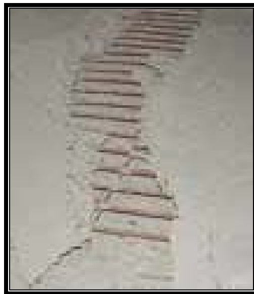
Figure 6-14. Concrete Slabbing
