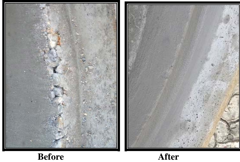
Figure 3-2. Form Bleed Repair – Acceptable
