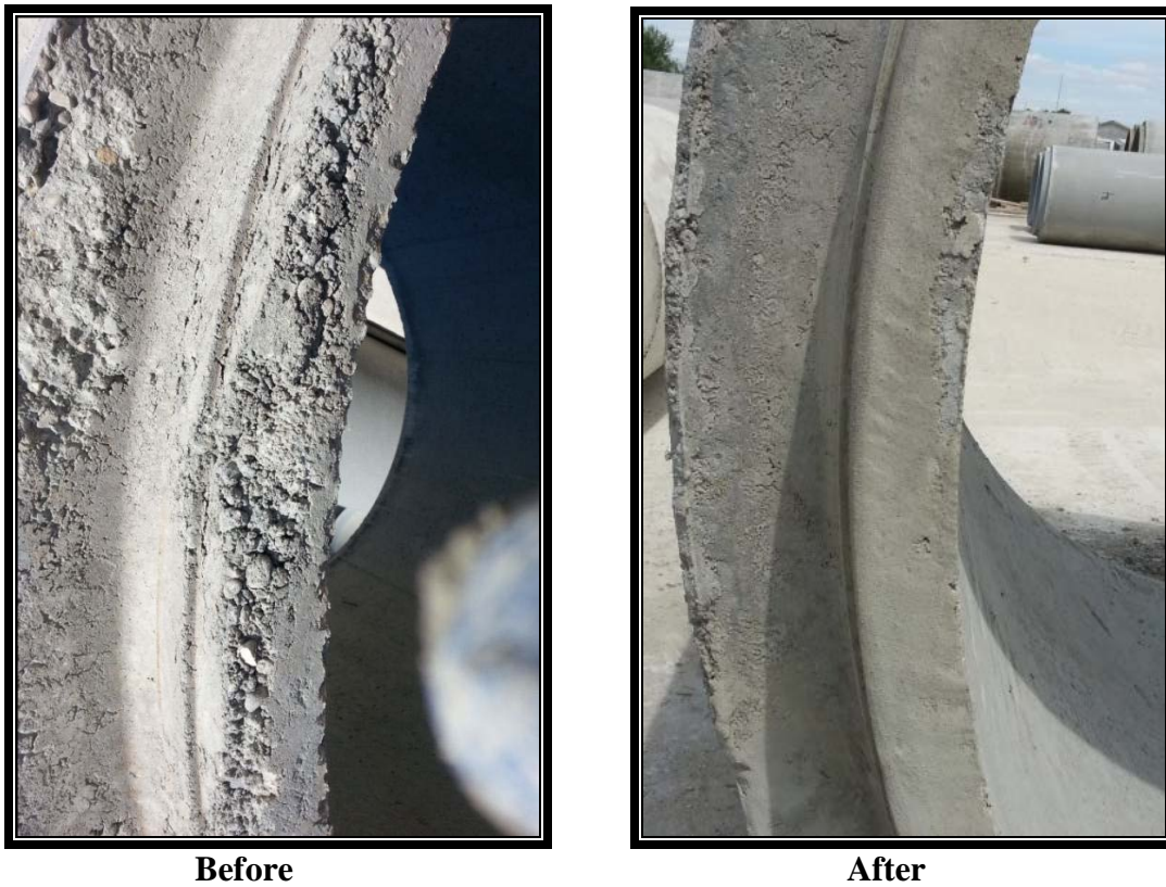
Figure 2-11. Pipe Spigot Repair - Acceptable
