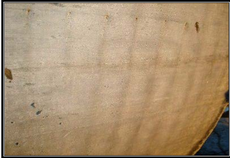
Figure 4-1. Wall Shadowing – Not Acceptable
