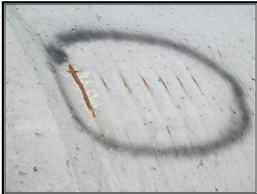
Figure 4-2. Wall Shadowing – Not Acceptable
