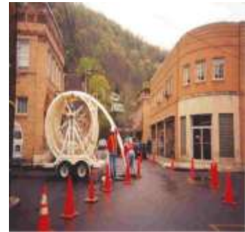
Figure 2-5. HDPE FnF Being Inserted in a Pipeline
