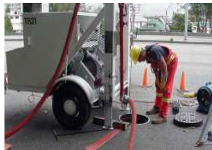
Figure 2-7. Winching Liner in Place
