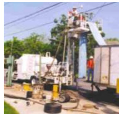
Figure 2-1. Inversion Set-Up
