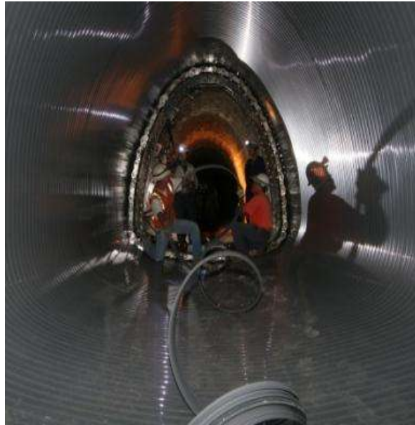
Figure 2-13. Machine Wound in Place Liner System
