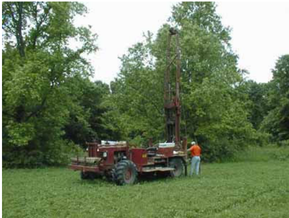
Figure 1. Off-road drill rig.
