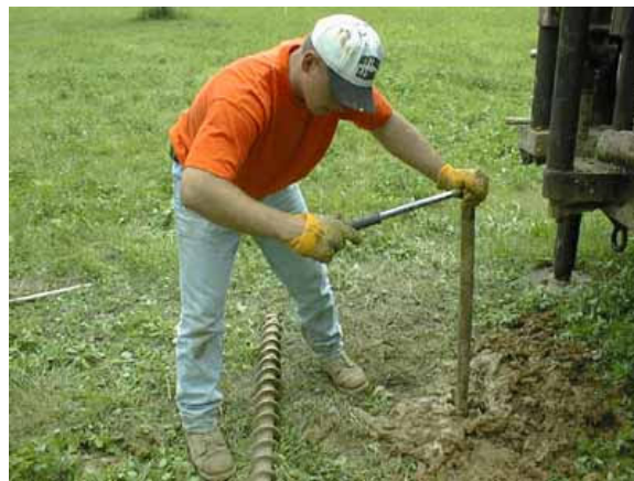
Figure 17. After allowing the shear vane to sit in the soil for a few minutes, the driller uses a torque-wrench to apply torque to the shear vane shaft. When the shear vane reaches maximum torque (indicated when shaft begins to rotate), the torque is recorded.
