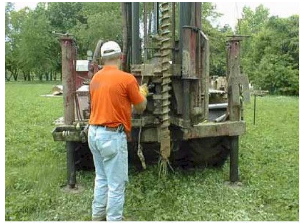
Figure 2. Operator prepares to use 3- to 4-inch diameter continuous-flight auger.
